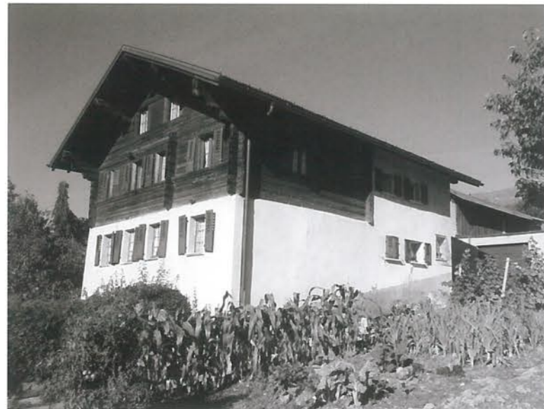
The house before renovation. Photo Savioz Fabrizzi Architectes
