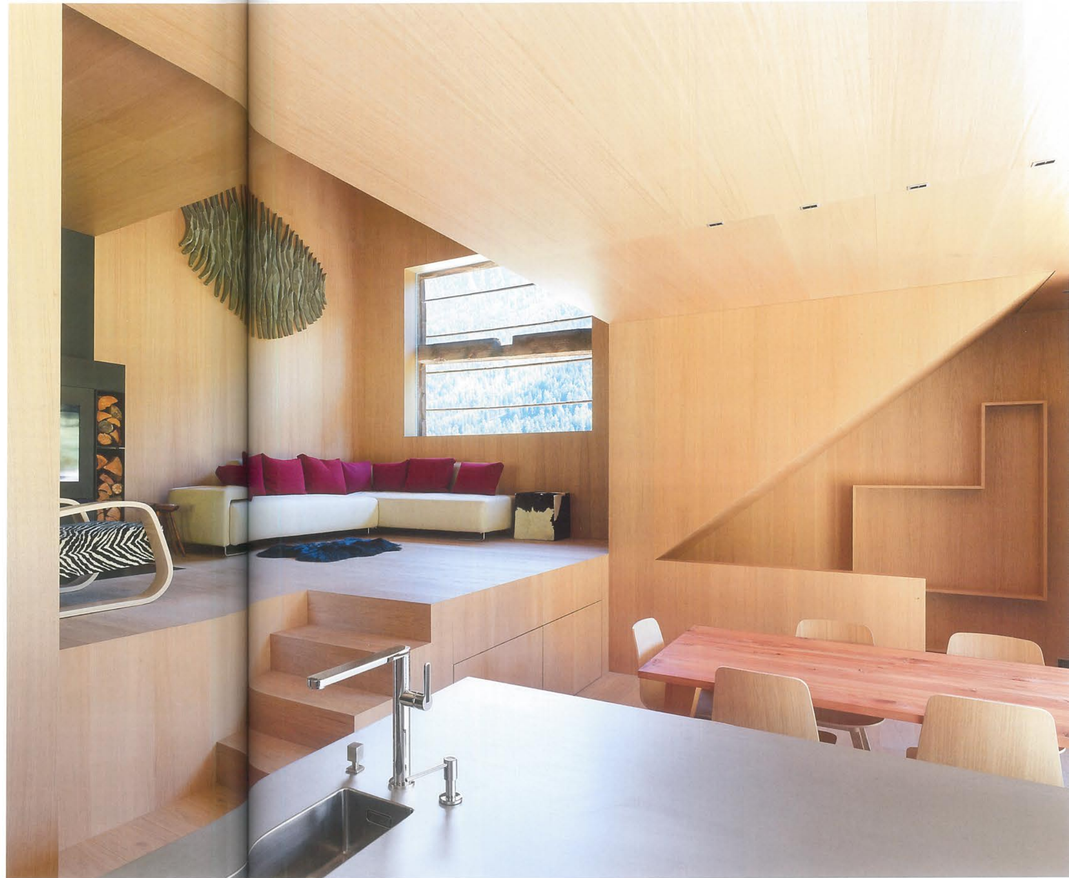
The new internal skin of the barn consists of oak panels.
