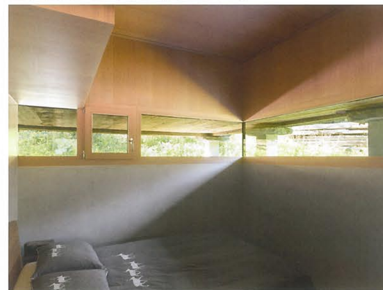
A band of glazing between base and superstructure enables natural light to reach the bedrooms in the basement.
